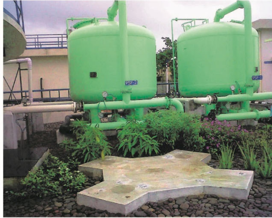
Pressure Sand Filters
